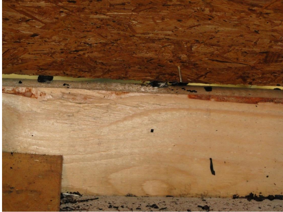
Figure 4. Trapped embers in the fascia-to-roof sheathing gap.
