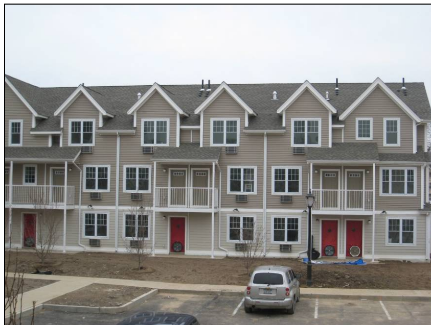
Sleeve AC Systems in a Staten Island Townhome Project
