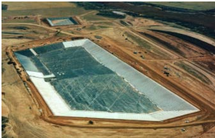
Figure 60. Aerial view of the double composite liner system at the base of the Monticello mill tailings repository
