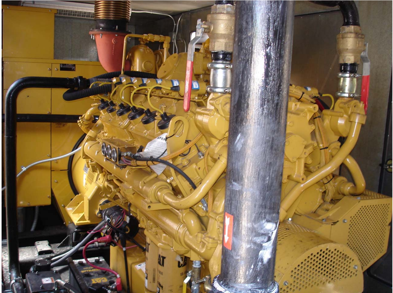
Caterpillar Engine Generator (G3412C)
