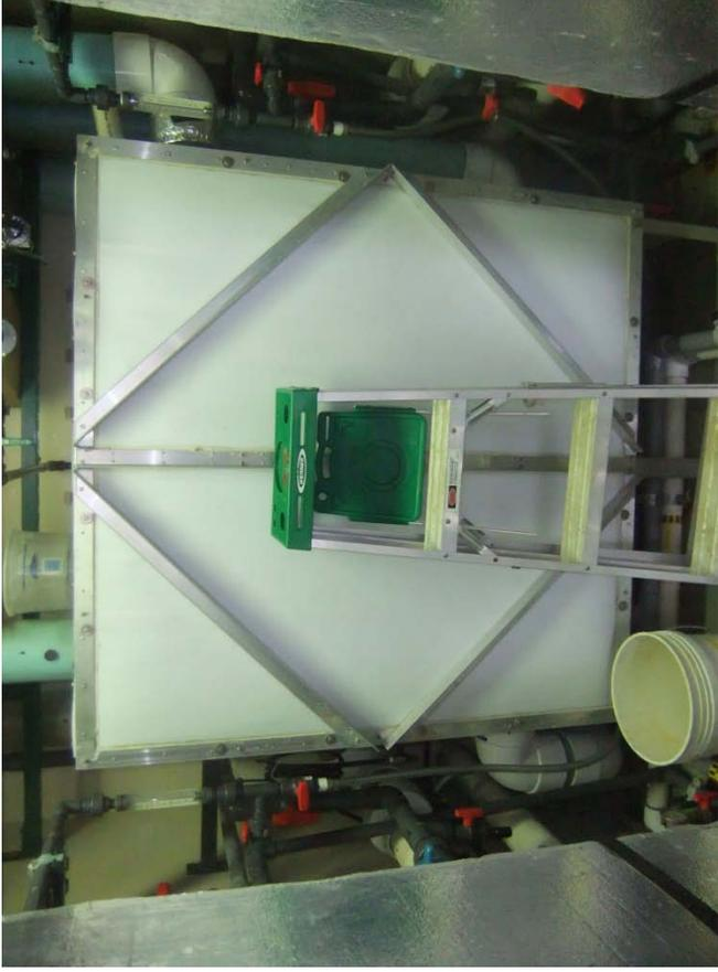
Heat exchanger, constructed of same material as treatment towers, to pre-heat inlet air and cool saturated outlet air (water condensing out of outlet air in heat exchanger is collected)
