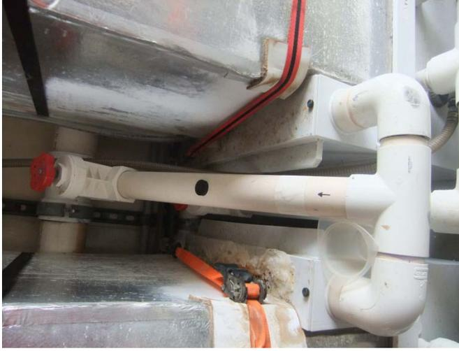
Pipes carrying saturated air from the system and tanks collecting treated water at the side
