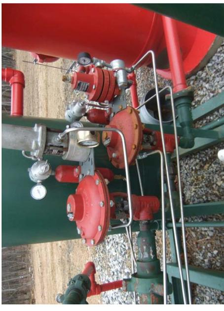
Series of control valves used to reduce pressure before feeding to the production pipeline
