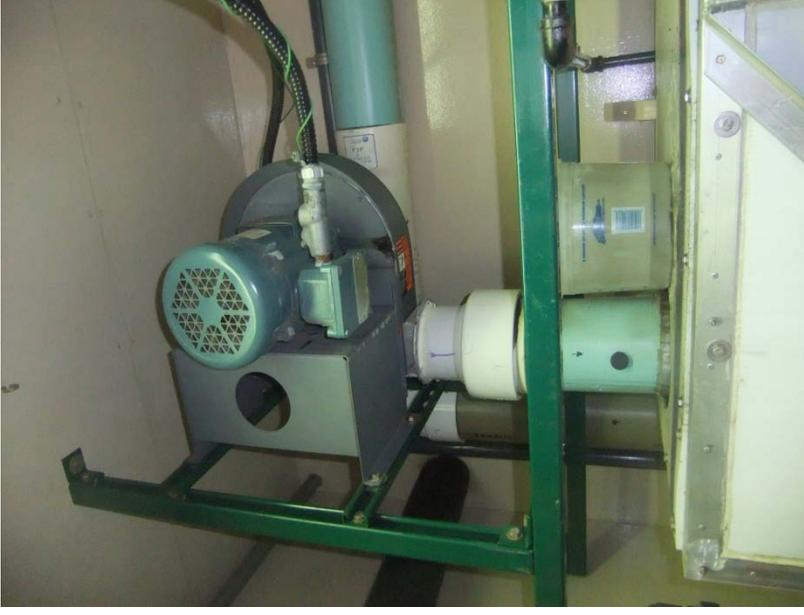
Blower drives air flow through heat exchanger
