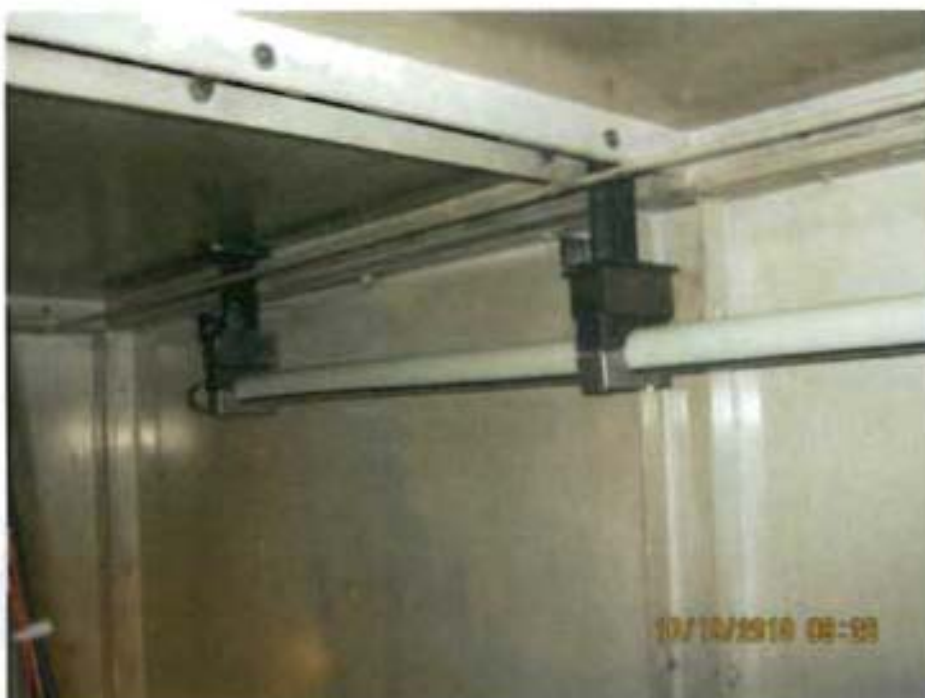
Fire Foe™ tube installed with brackets (rear half)
