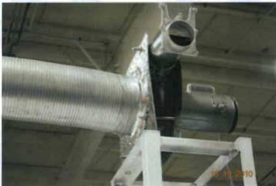
Exhaust duct and blower assembly
