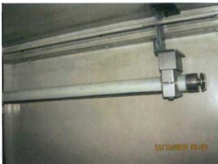
Fire Foe™ tube installed with brackets (front half)
