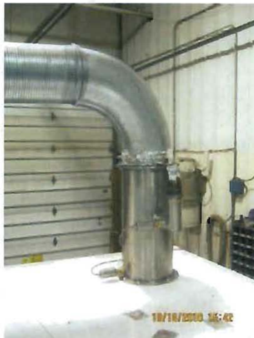
Roof view of exhaust duct. The lower stainless steel section housed the HEPA filter
