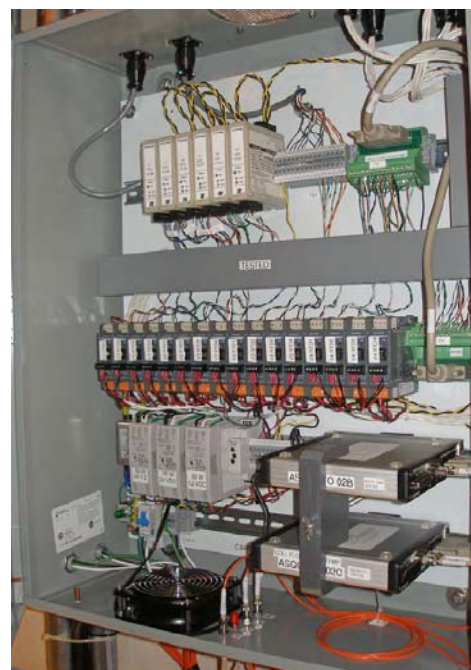
Figure 23. The analog interface box, Box 4, contains two ASQUIRT02 units to echo water cooling information to both PLC and TPS.
