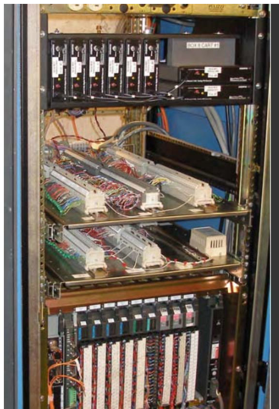
.....but with considerable wiring overhead, shown on the two trays between the Box 8 rack and the PLC.
