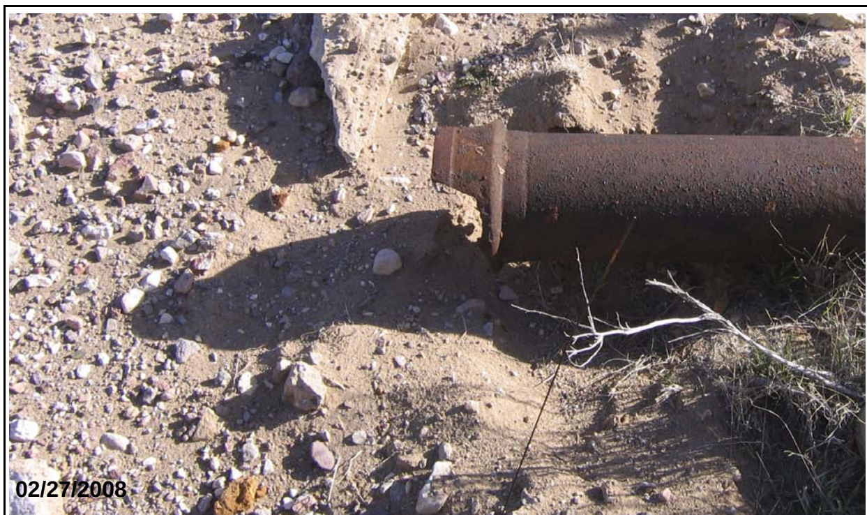
Figure A.11-4 Contaminated Pipe Waste Dump CAS 25-23-21, Radioactive Waste Dump
