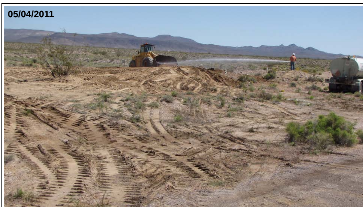
Figure D.1-11 CAS 25-23-21, Radioactive Waste Dump, Leveling of Soil Piles
