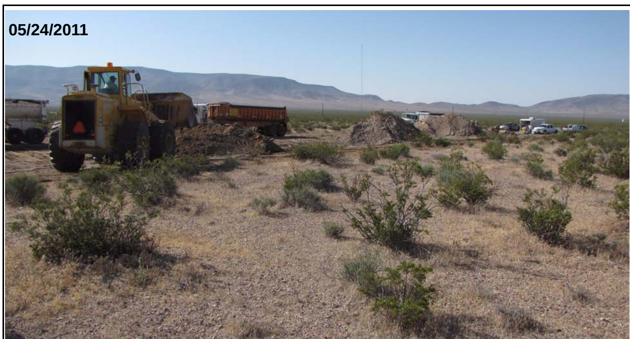
Figure D.1-8 CAS 25-08-02, Waste Dump, Debris Piles Being Loaded Out
