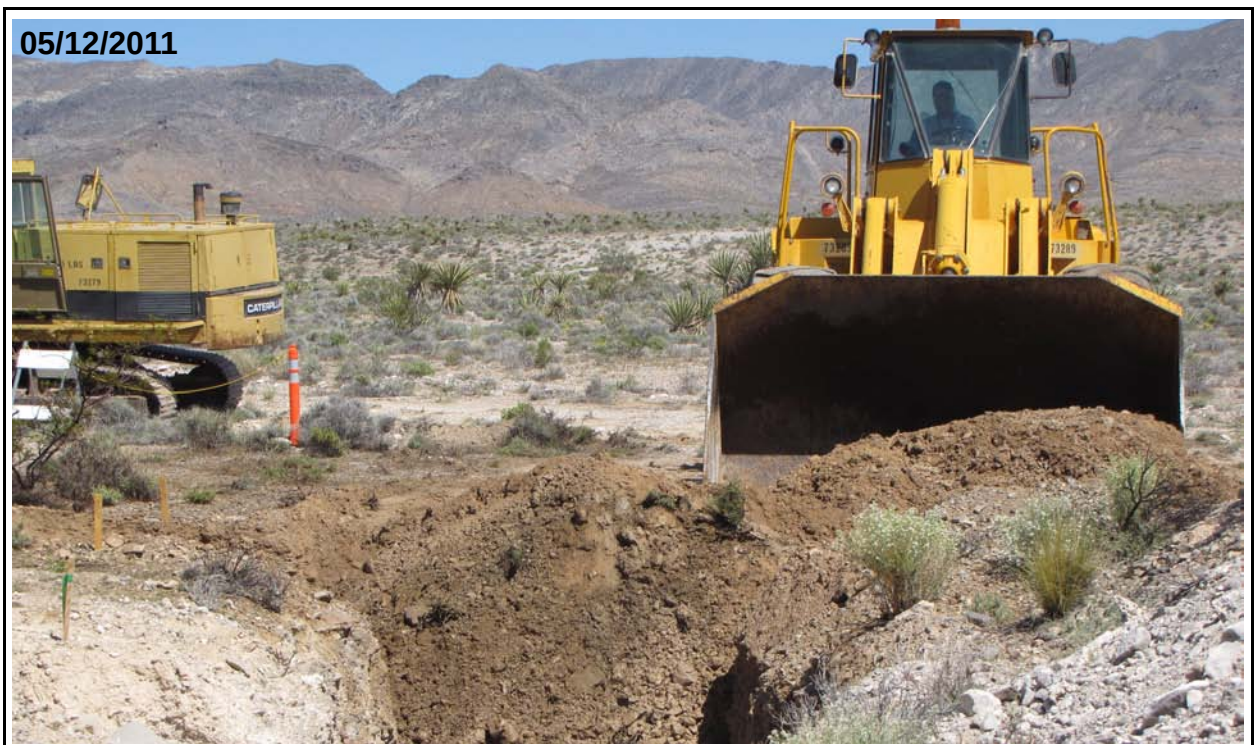
Figure D.1-5 CAS 23-21-04, Waste Disposal Trenches, Front-end Loader Backfilling Trench
