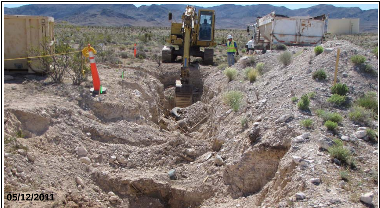
Figure D.1-4 CAS 23-21-04, Waste Disposal Trenches, Debris Removal from Trench 3
