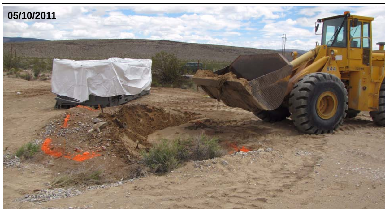
Figure D.1-12 CAS 25-23-21, Radioactive Waste Dump, Excavation of RMA, Soil Disposed of in Lined Intermodal
