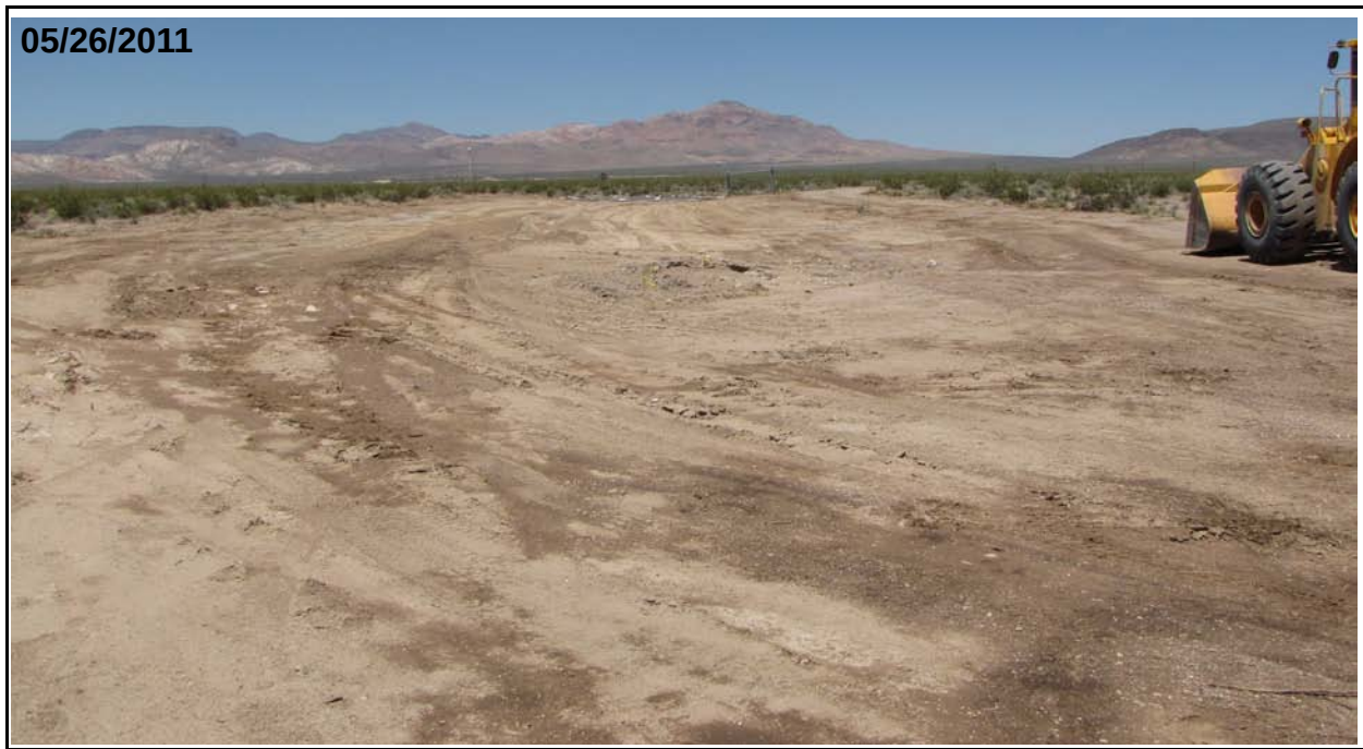
Figure D.1-9 CAS 25-08-02, Waste Dump, Debris Piles Removed
