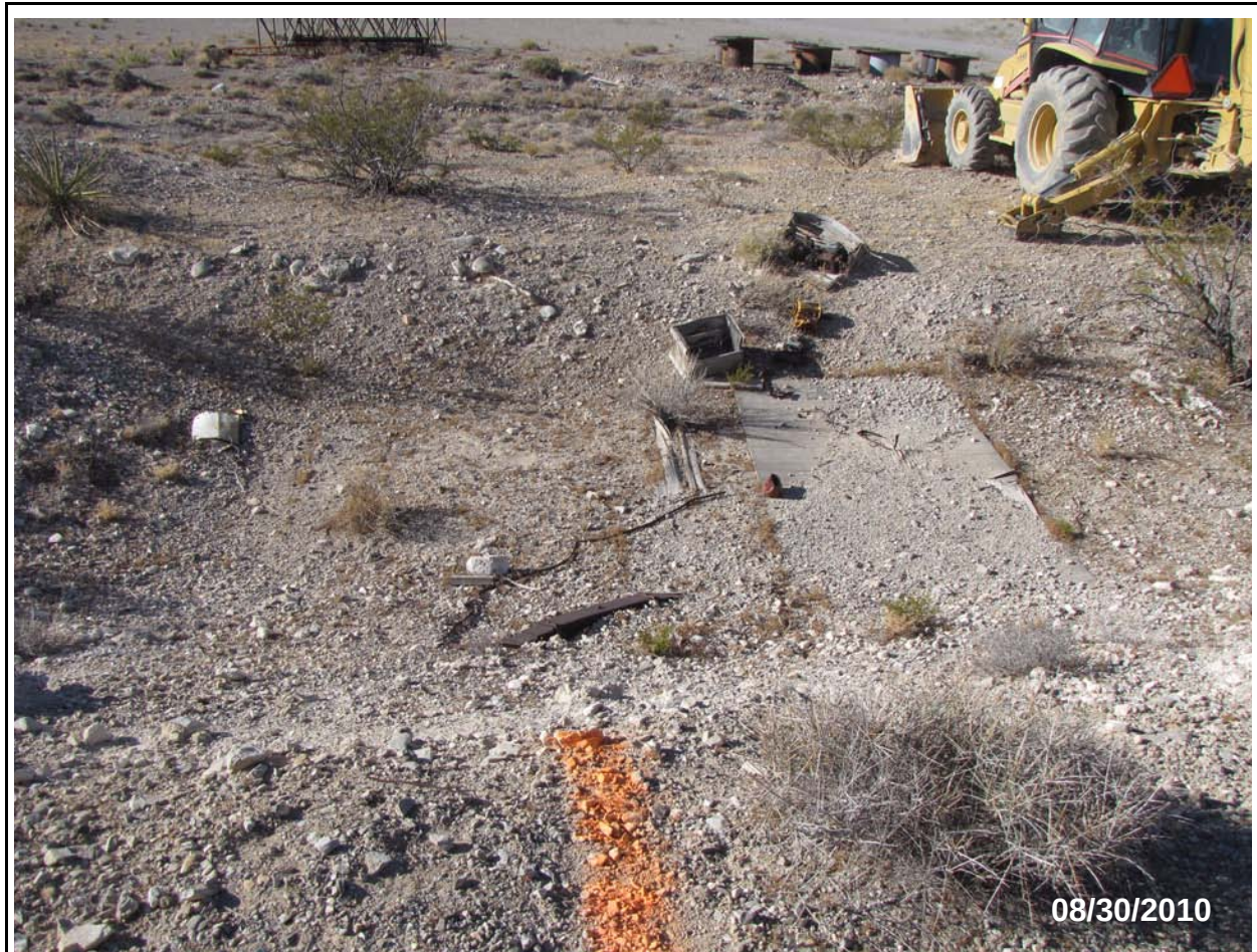
Figure A.9-2 Debris in Trench 6, Pre-excavation CAS 23-21-04, Waste Disposal Trenches
