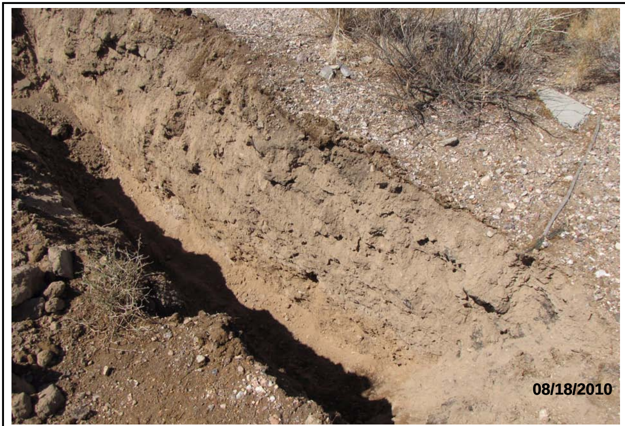
Figure A.12-3 Asphalt and Stained Soil in North Trench CAS 25-25-19, Hydrocarbon Stains and Trench
