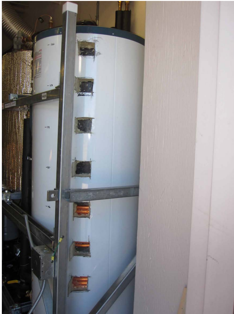
Figure 14. Location of external wall temperature sensors.
