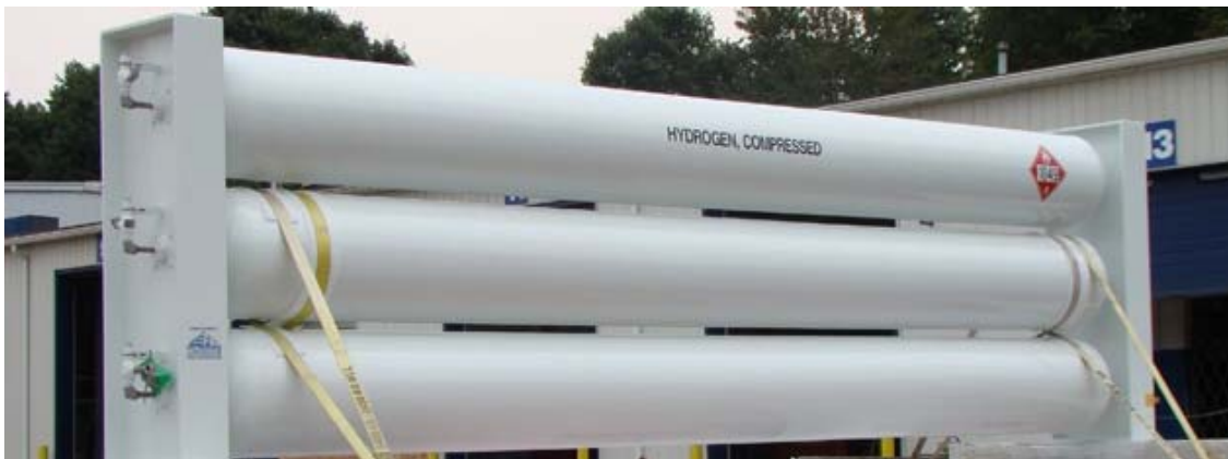
Figure 66 - Gas storage array for Demonstration System
