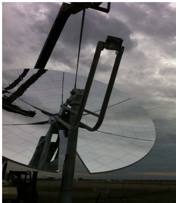
Figure 50 – Solar Dish Being Lifted Into Place
