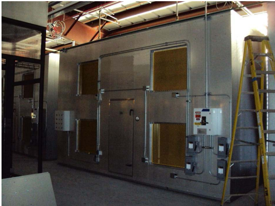
Figure A-4 Yahoo! Compute Coop's Skid-Based Cooling System – Lockport, NY
