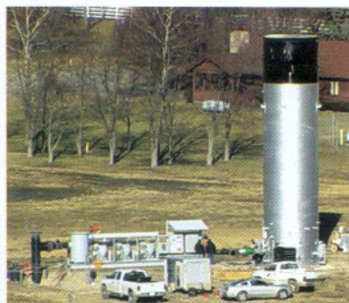
While the flare (at right above) is the Maximum Achievable Control Technology required for collected landfill gas, SWACO wanted to go beyond that level of compliance and recover energy and fuels.
