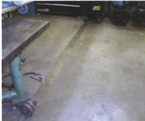
Figure 5. Welding cables placed in a concrete groove, covered by a stainless steel plate.
