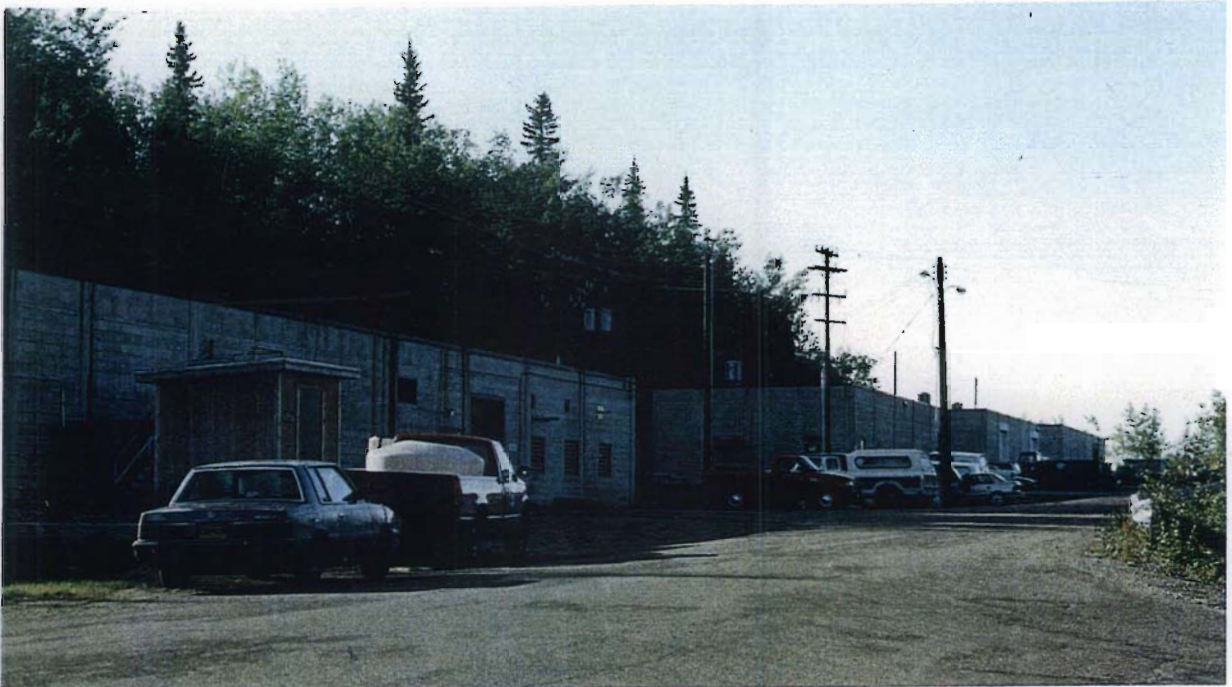
FIGURE B.5. Engineer Hill Munitions Facility, SS56. Location is at the upper road showing the maintenance and operations buildings. The water supply well is located at the concrete pad immediately left of the small wooden shed (Bldg 6156)
