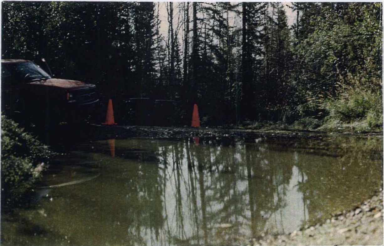
FIGURE B.6. The Leach Field Crib at the Bottom of Engineer Hill, SS56. Road is the old access to Lily Lake. At the time of the photo (August 1993), water was seeping out of the embankment at the left and forming the standing pool. Well 56M03 is located under the safety cone, to the right of the cuttings drums.
