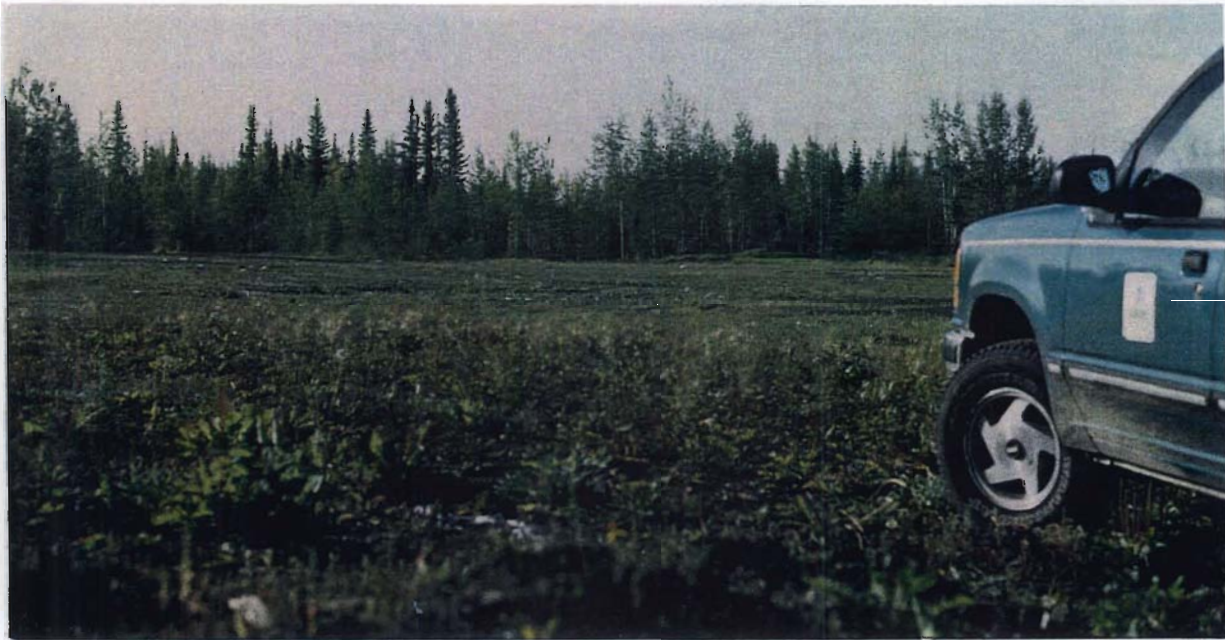
FIGURE B.3. Snow Disposal Area at LF02. The graded surface is the cap for the landfill
