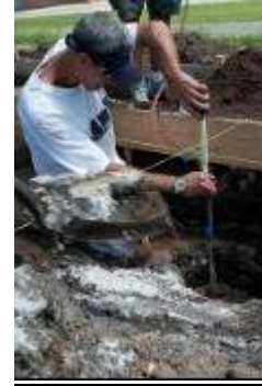
Figure 2-5. FSEC's John Sherwin measures for exact depth placement. Yellow strings mark top of slab.
