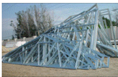
Figure 3-44: Steel trusses produced on site
