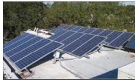
Figure 3-29: 2.25kWp Photovoltaic power system on roof top of 2007 TNAH
