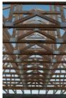
Figure 2-7. Rafter design allows for a walkway above insulation level for easier attic walking for experiment changes.
