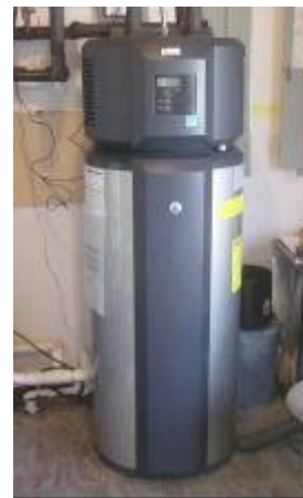
Figure 2-41: Commercially available heat pump water heater
