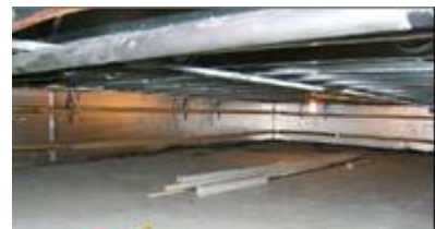
Figure 3-13: Weather tight and insulated crawlspace
