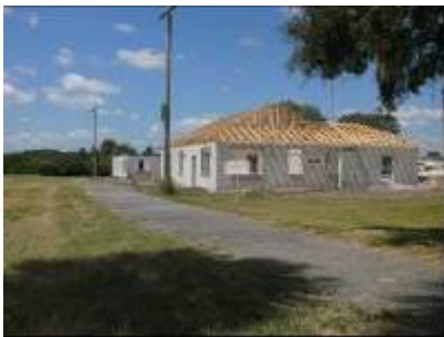
Figure 2-6. Rafters were placed on the East house by hand. West house shown without rafters in background.
