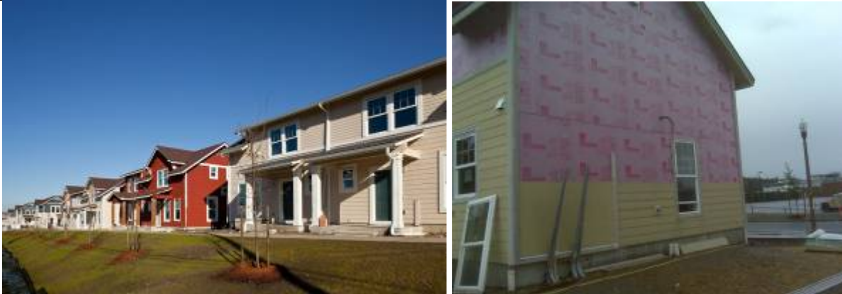
Figure 8 – Salishan 7 (L) and foam sheathing detail on demonstration unit
