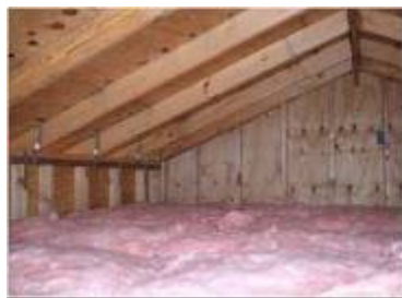
Figure 2-51: Conventional Shed with Vented Attic and R-30 Fiberglass
