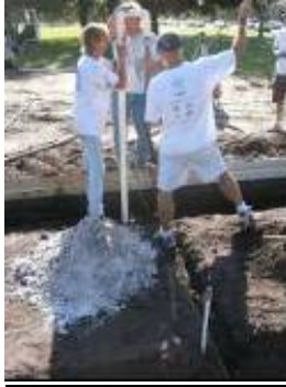
Figure 2-3. Well is dug using water.
