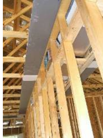
Figure 4-7: Innovative interior duct system design shown in plan at left (shaded areas) and under construction at right. Note that the ceiling of the duct chase that forms the attic air barrier is installed above the top plates, significantly reducing the number of drywall joints that need to be sealed. This detail resulted from a collaboration between Ken Fonorow of FL HERO and the sub-contractors involved in the construction of the chase.
