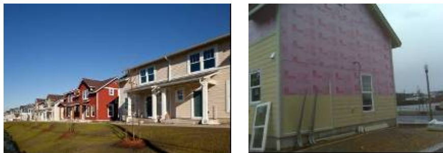
Figure 4-12 – Salishan 7 (L) and foam sheathing detail on demonstration unit
