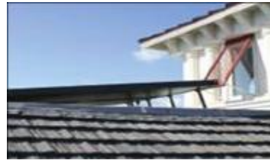
Figure 3-23: Solar water heater on TNAH 2008
