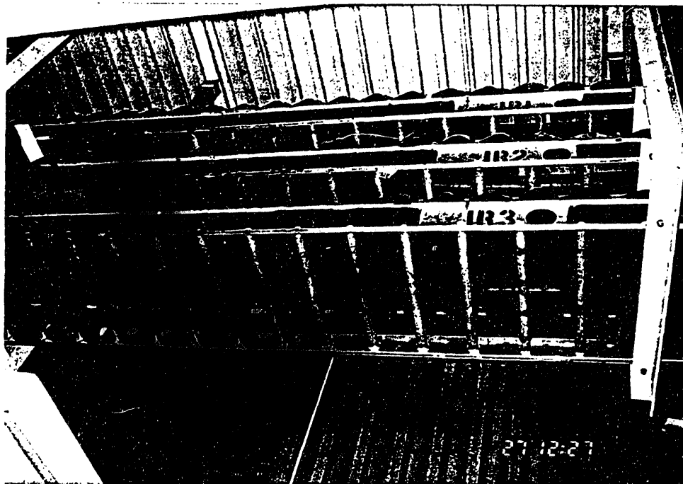
Figure 5.2-8: Trapeze Supported Cable Trays
