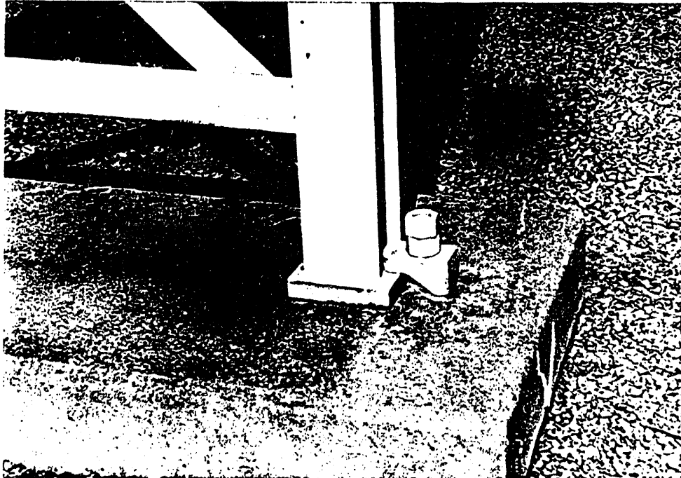
Figure 5.2-18: Friction Clip at the Base of Steel Frame Supporting Circuit Breakers
