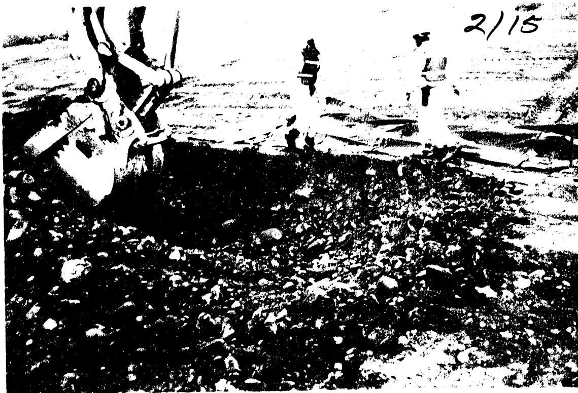
TP M-CF-20. Beginning excavation. Note one inch of tailings on the surface.
