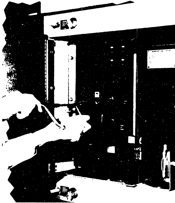
Figure 3-16. Worm-Gear Circuit Breaker Racking Mechanism, Westinghouse Low-Voltage Circuit Breaker, Types DS and DSL.[3.8]
