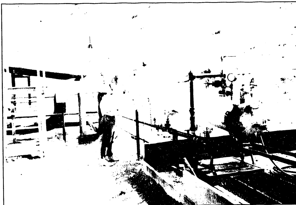
Lynn Endsley working at the gas line pig launcher at Naval Petroleum Reserve No. 1.
