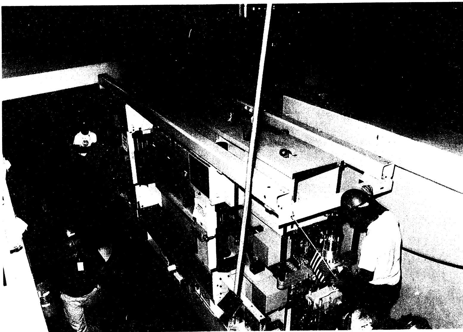
Figure 9. The first ALS U5.0 undulator was installed in the storage ring on May 7 with only inches to spare. The 4.55-meter magnetic structure along with its support structure, a combined weight of nearly 25 tons, was lowered into the ring after parts of the concrete shielding were removed. The second U5.0 was installed in June.
