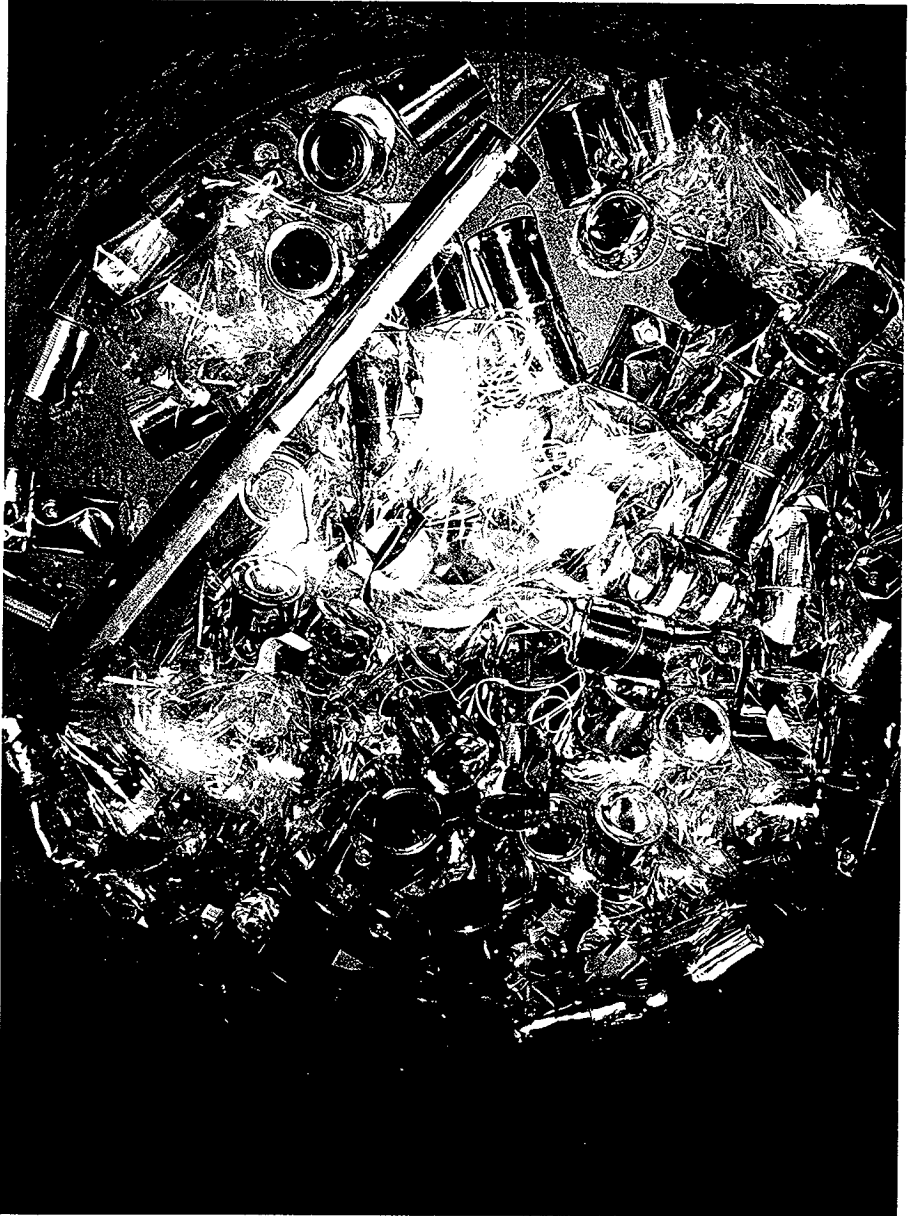
Figure 2-25: Condition of Waste Containers in Caissons (200 Area)
