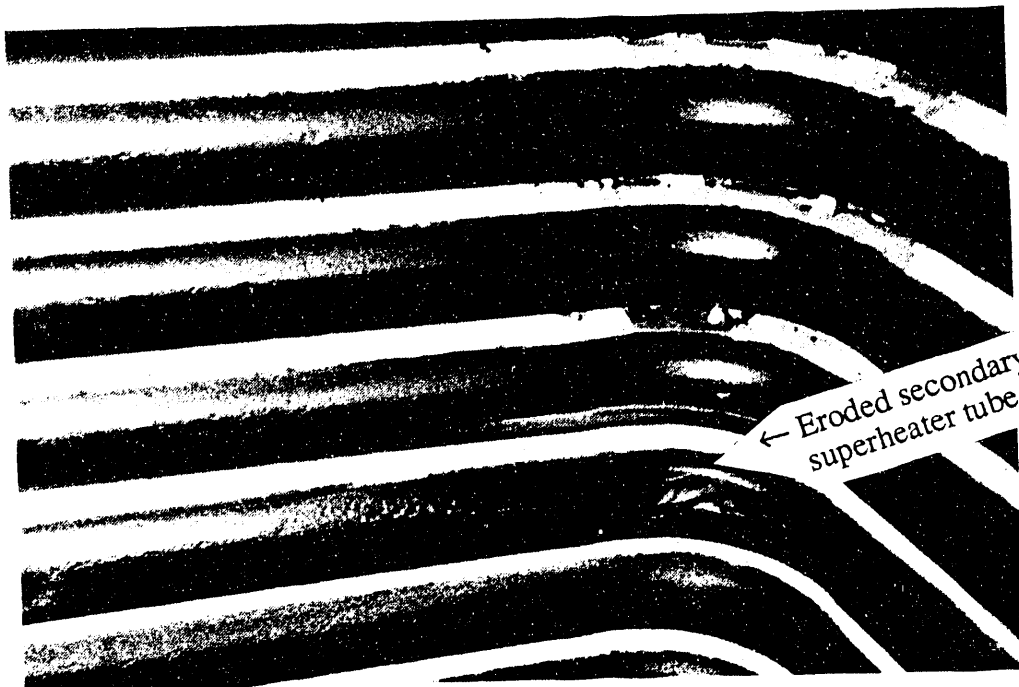
Figure 13-16. Eroded Secondary Superheater Tubes in Combustion Chamber Corner.
