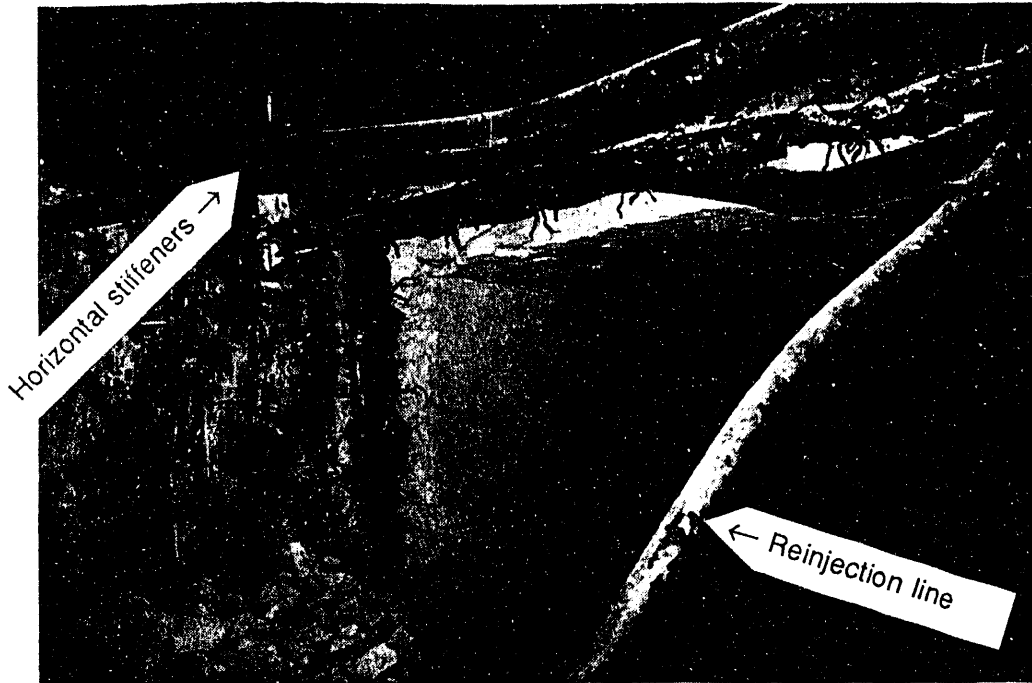
Figure 13-3. Distortion of the Windbox Horizontal Pipe Stiffeners and Reinjection Line.
