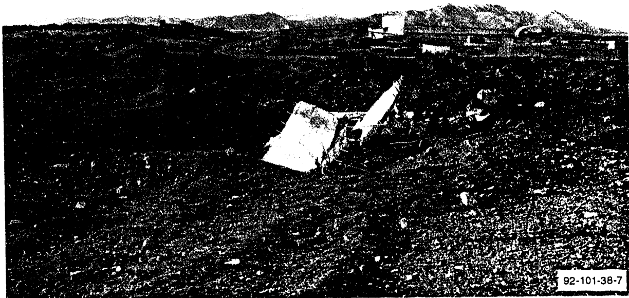
Figure 31. View of remaining pieces of concrete foundation prior to completion of backfilling turbine building site.
