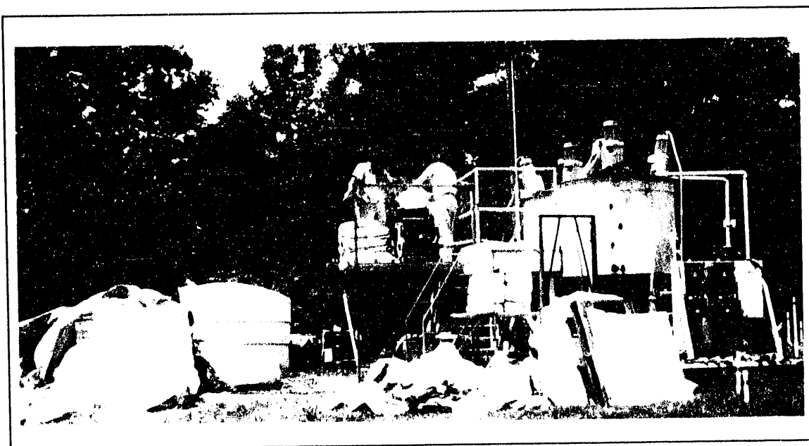
Fig. 27. Preparation of the grout formulation using a cyclonic mixer and grouting unit at the field site (ORNL 7096-91).
