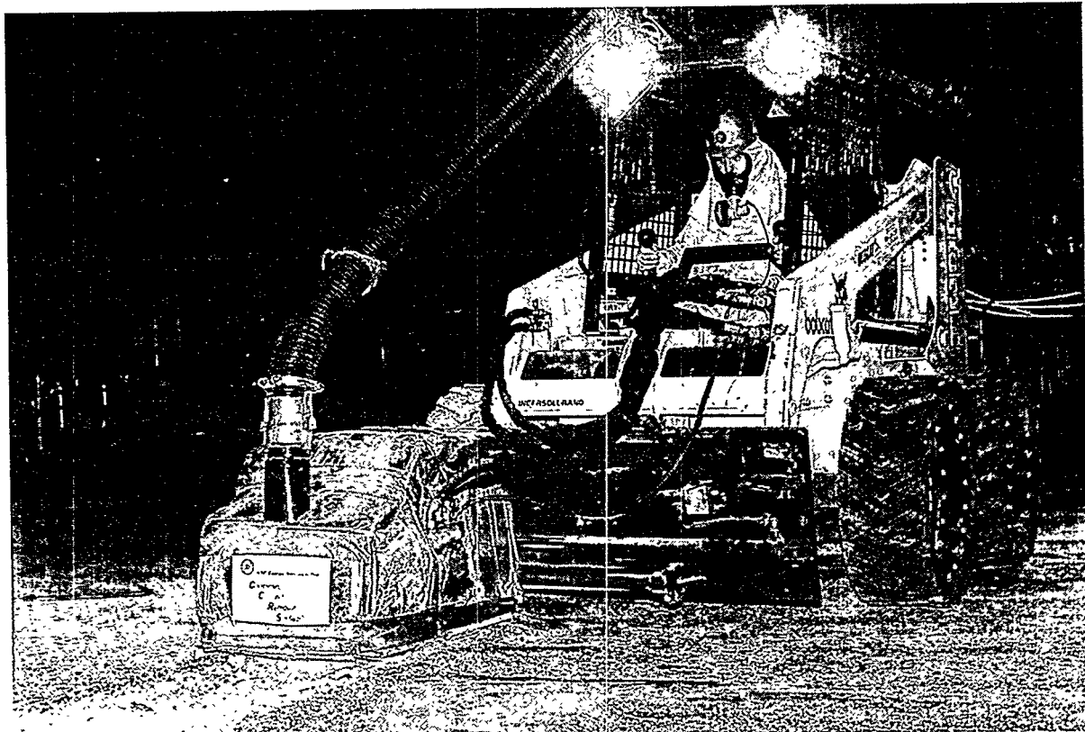
Figure 10. Rotary drum planer operating in Fernald's Plant 9.
