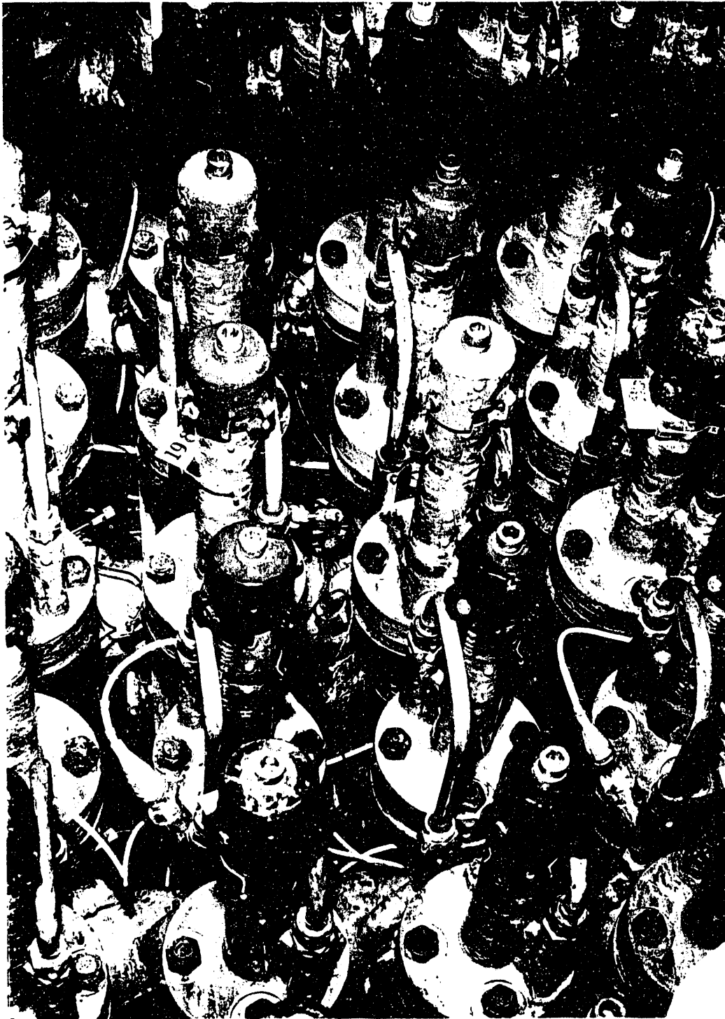
EXHIBIT NO. 11 105-H REAR FACE - VIEW SHOWING WET CONDITIONS, SCALE BUILDUP, THERMOCOUPLE CONNECTIONS LOOSE FROM VIBRATION
