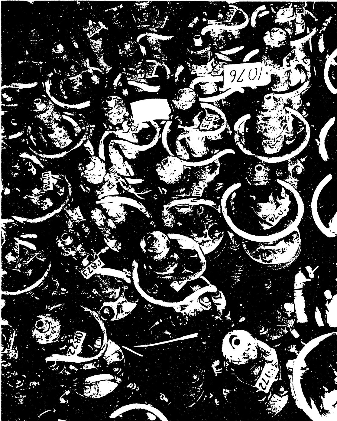
EXHIBIT NO. 9 105-F REAR FACE - VIEW SHOWING SCALE BUILDUP
