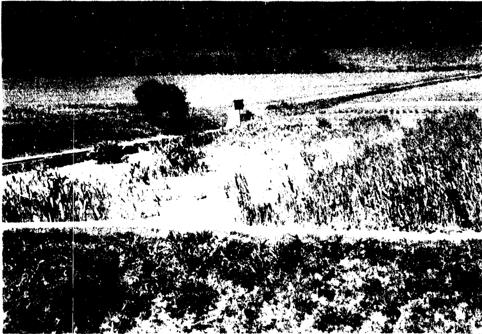
The See, West Germany, EHTS site is divided into two zones, one with water ponded at the soil surface and the other in which water flows only underground through the root zone.
