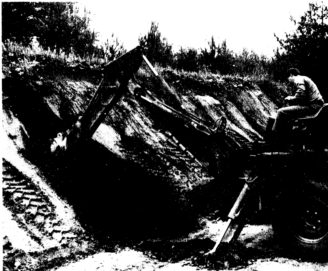
FIGURE 6 Excavation of the Trench in the Berm at Range 124 at GTA during July 1992
