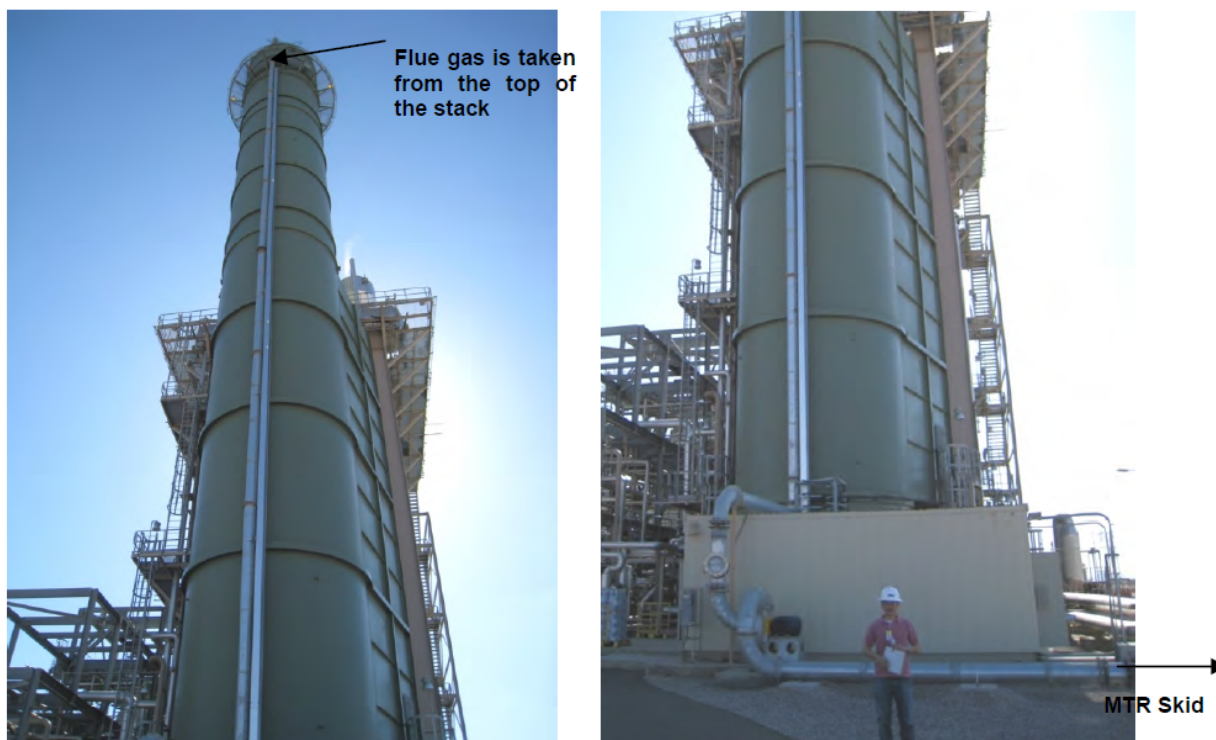
Figure 4-14. Stack from which Flue Gas Is Directed towards MTR CO 2 Membrane Skid
