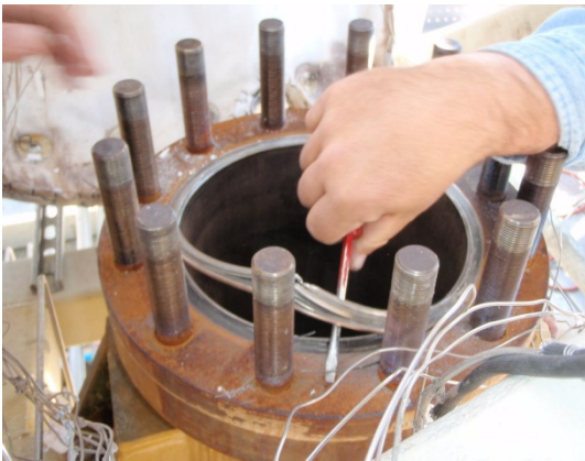
Figure 3-27 . Taking Out the Worn Gasket
