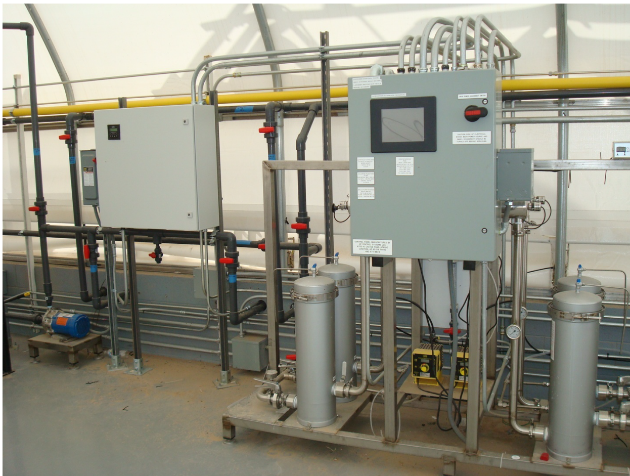
Figure 4-13. Water Treatment Filtration Skid with Control Panels
