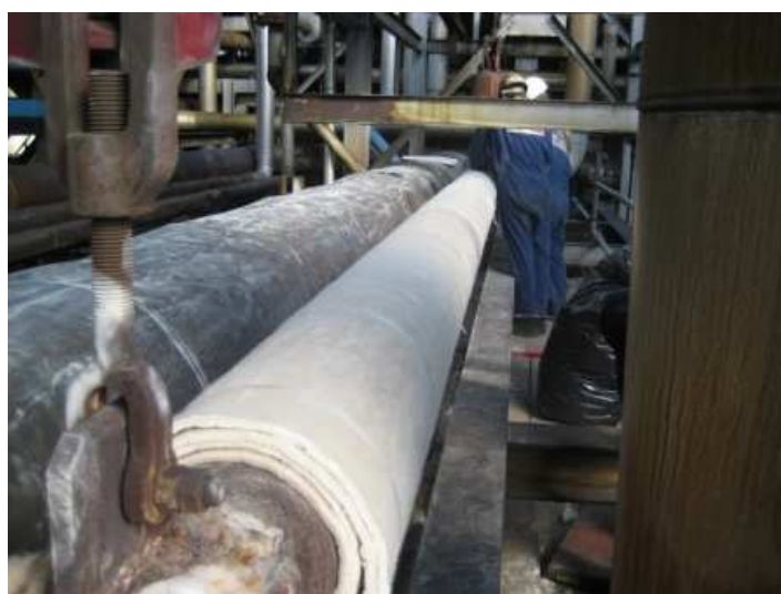
Figure 37. Pyrogel installation on straight section.
