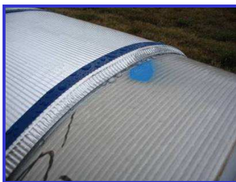
Figure 22. Crimped and Sealed Edges
