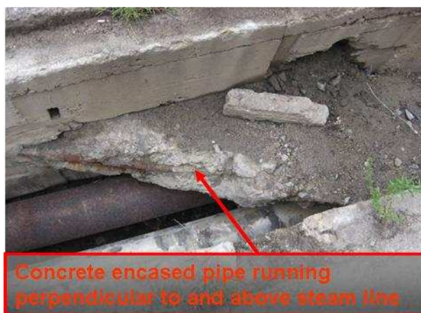
Figure 28. Pipe obstructions encountered in the trench such as this intersecting water line.
