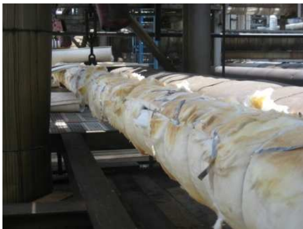
Figure 36. Installation site with pre-existing mineral wool insulation still on the pipe.
