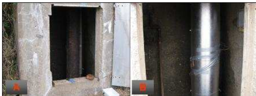
Figure 30. Pipe section (A) before and (B) after application of cellular glass
