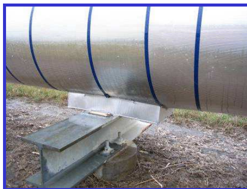
Figure 23. Insulated Pipe Support
