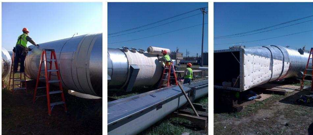
Figure 34. Installation of Pyrogel XT on various sections of ductwork.
