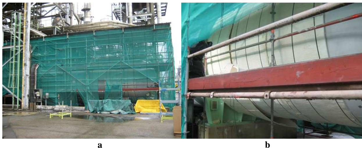
Figure 41. Installation of Pyrogel XT on “bullet” tank at Port Jerome Refinery: a) full tank image and b) close up of aerogel installation in progress.
