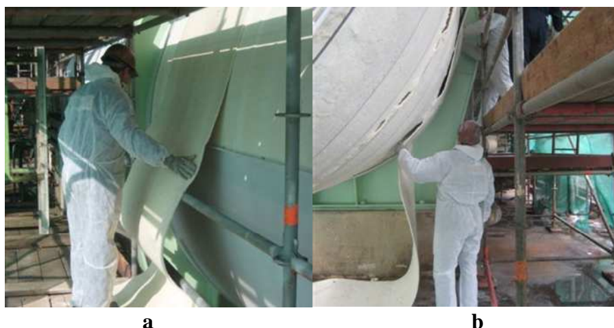
Figure 42. Workers installing Pyrogel XT on a bullet tank: a) top half, b) bottom half.
