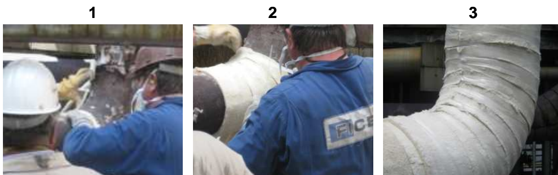
Figure 38. Fitting a lobster tail elbow section on a 90° elbow at Port Jerome.
