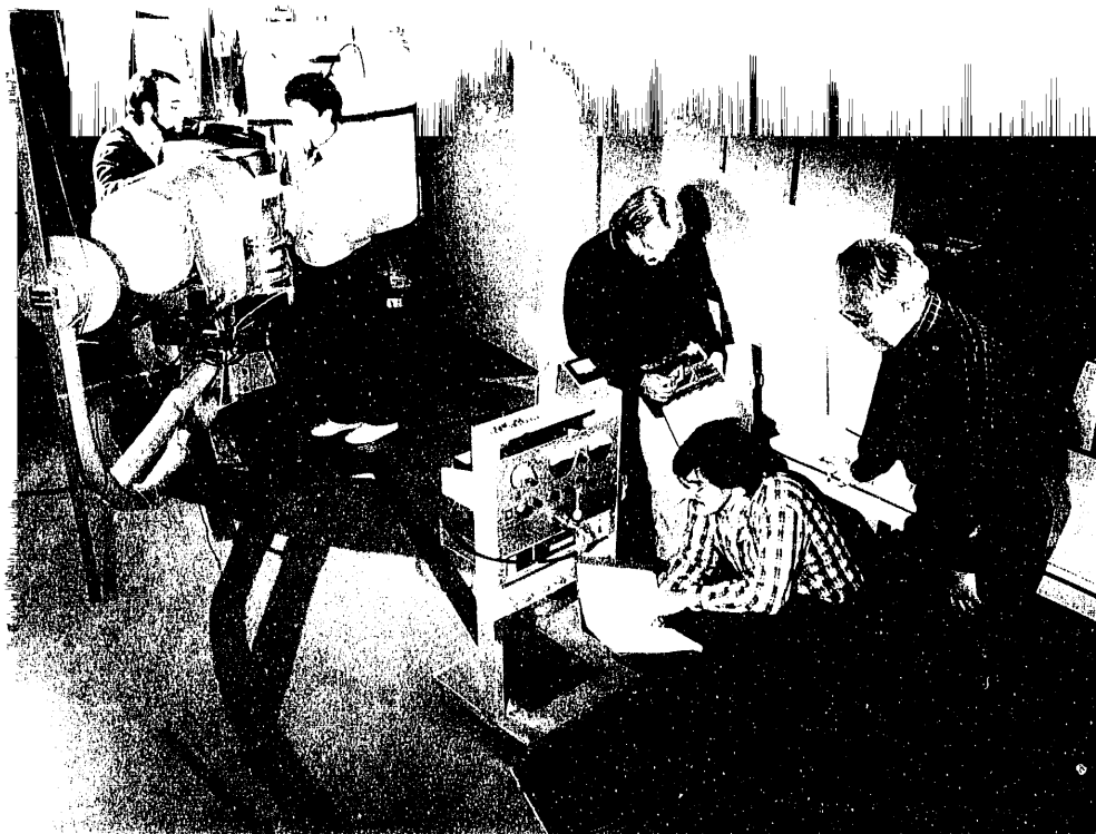
Figure 26. At the H7 Spectrometer (from left) Bernhard Keimer (MIT) and Kazu Yamada (Tohoku University, Japan) are adjusting the spectrometer; Thomas Thurston (BNL) is pulling out a mask that will be used to define the neutron beam; and John Tranquada (sitting) and Gen Shirane (BNL) are checking the sample temperature. These researchers, along with Robert Birgeneau of MIT, are studying high temperature superconductors.
