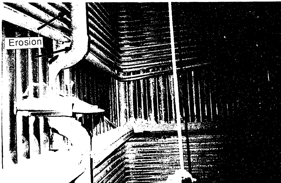
Figure 16-24. Secondary Superheater Shelf Arrangement and Erosion Locations Around Water-Tube Supports (February 1991 Outage).
