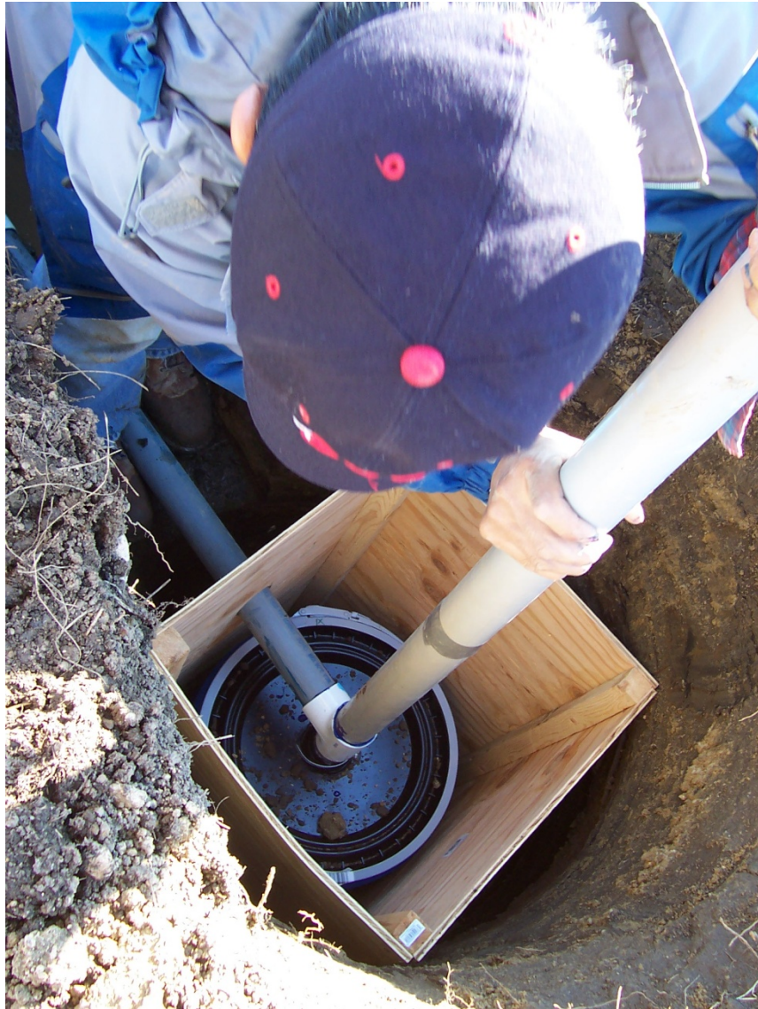
Figure A-7: Installing leachate collection tank.
