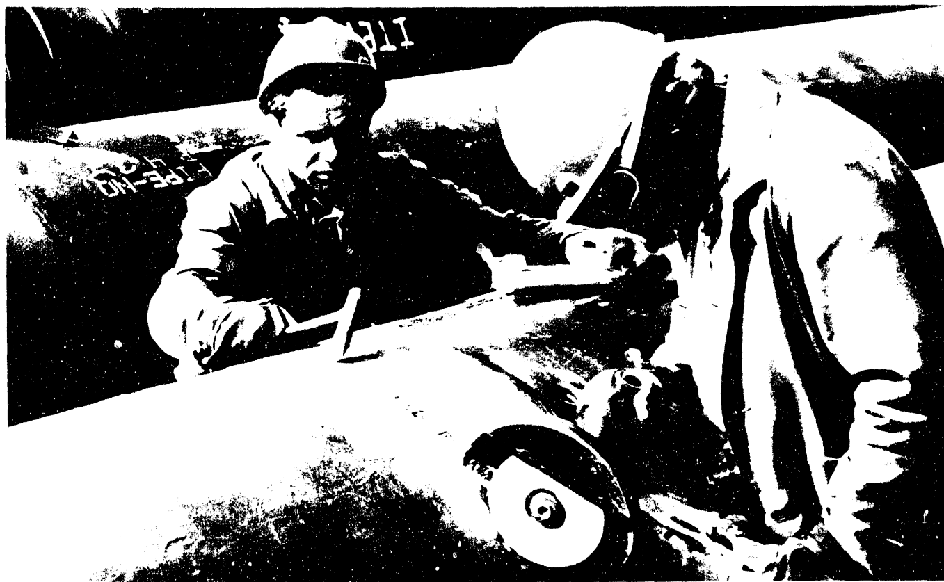
Welders grind seams on a 48-inch pipeline section, prior to installation.
