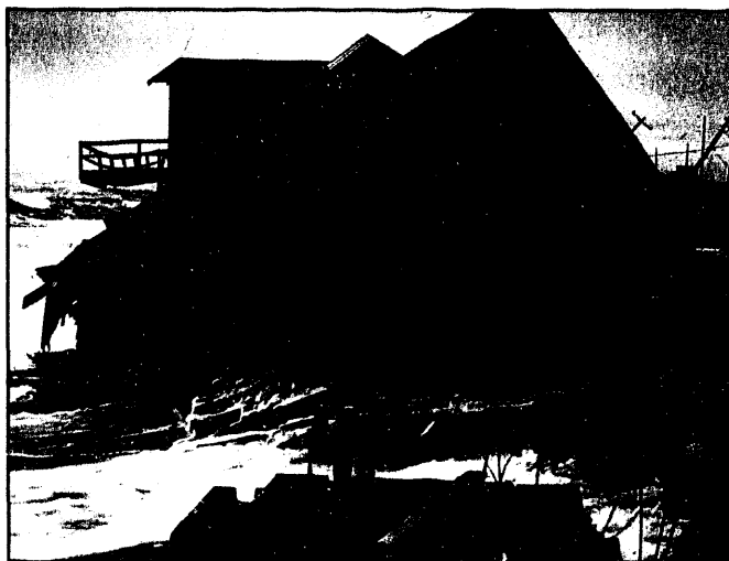
Winter storm damage, Kitty Hawk, N.C.
