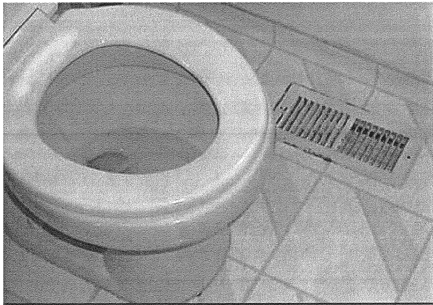
Figure A-4. Example of a register that is hard to access. The only way to measure flow at a register like this is by using a bag with a flexible wire coat hanger around its entry that can be formed into a shape to fit in the available space
