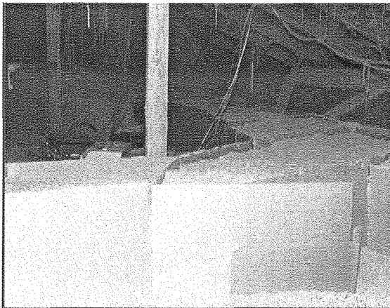
Blown –in insulation with cardboard forms
