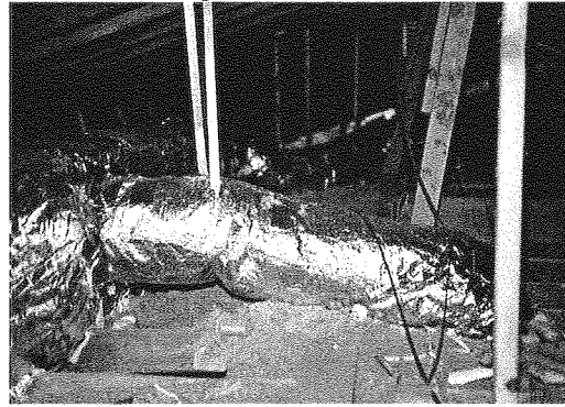
After adding duct insulation
