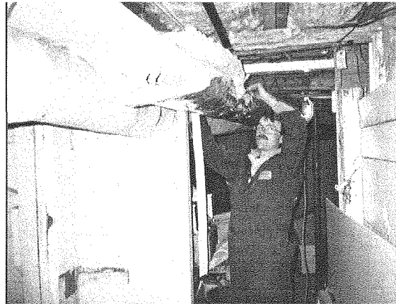
Installing Duct Wrap
