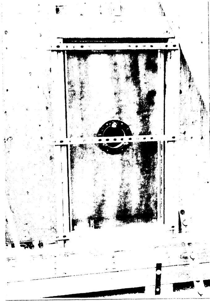
Photo 7 : Detail of sealed enclosure door and porthole
