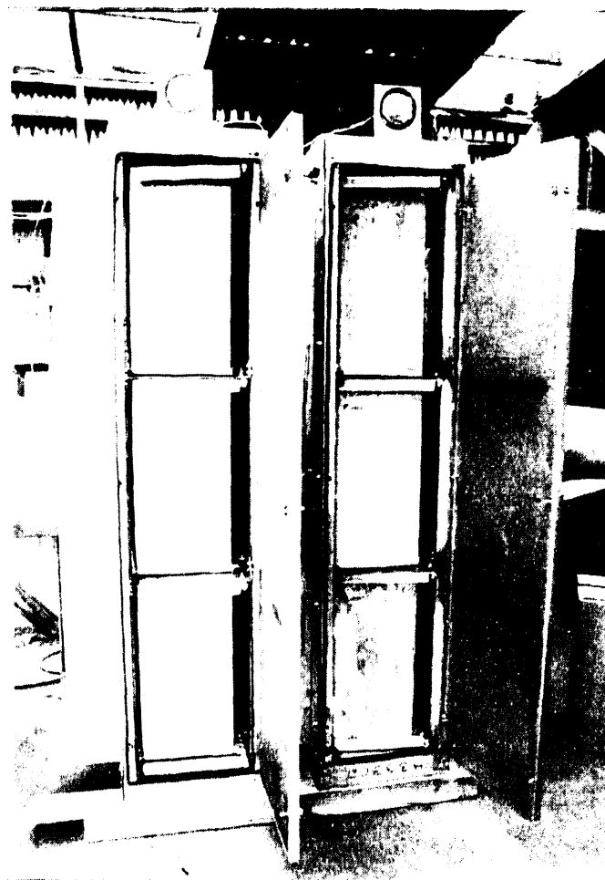
Photo 14 : Close up of pre-filters and HEPA filters
