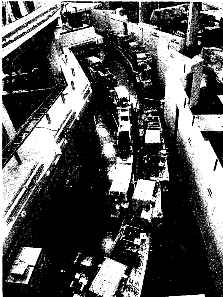
Figure 36. The booster-to-storage ring transfer line emerges from the injector-accelerator system cave on the left to meet the storage ring. Concrete shielding walls have been erected.
