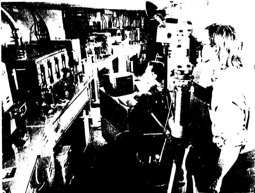
Figure 24. Precise surveying was required to position the booster girders.
