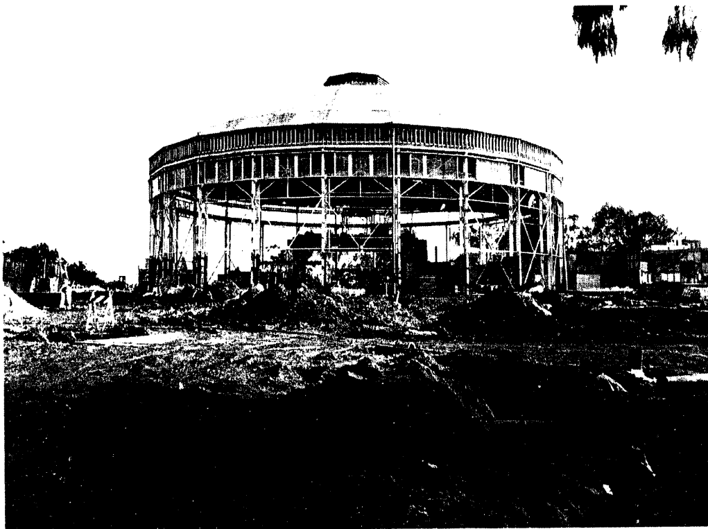
Figure 10. Beginning of ALS construction. The cyclotron dome has been incorporated into the new building.
