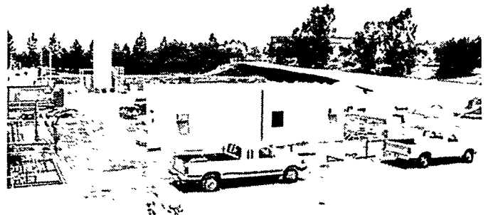
M-C Power 250 kW Fuel Cell Demonstration Plant UNOCAL Fred L. Hartley Research Center Brea, California Construction Phase 5/11/94
