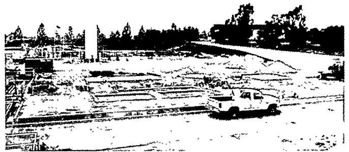
M-C Power 250 kW Fuel Cell Demonstration Plant UNOCAL Fred L. Hartley Research Center Brea, California Construction Phase 5/10/94
