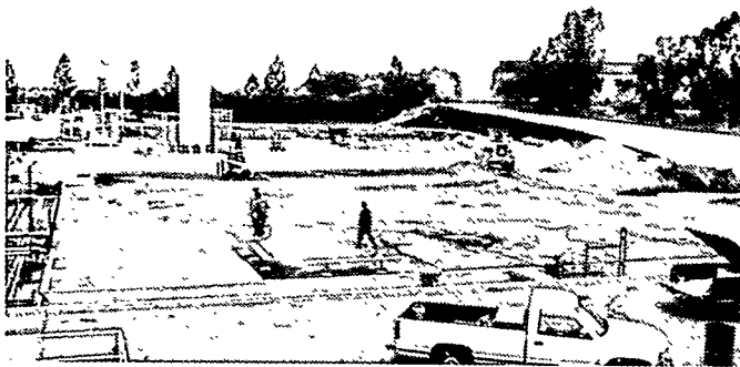
M-C Power 250 kW Fuel Cell Demonstration Plant UNOCAL Fred L. Hartley Research Center Brea, California Construction Phase 4/4/94
