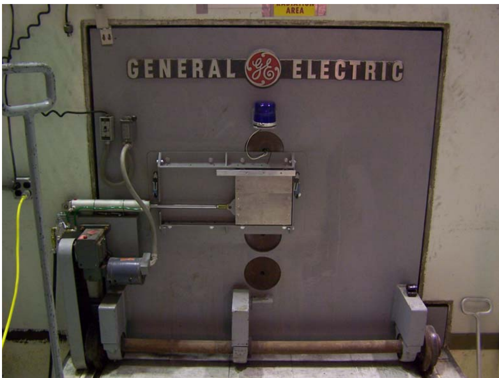
Figure 4. Beam shutter on the thermal column door (east view).
