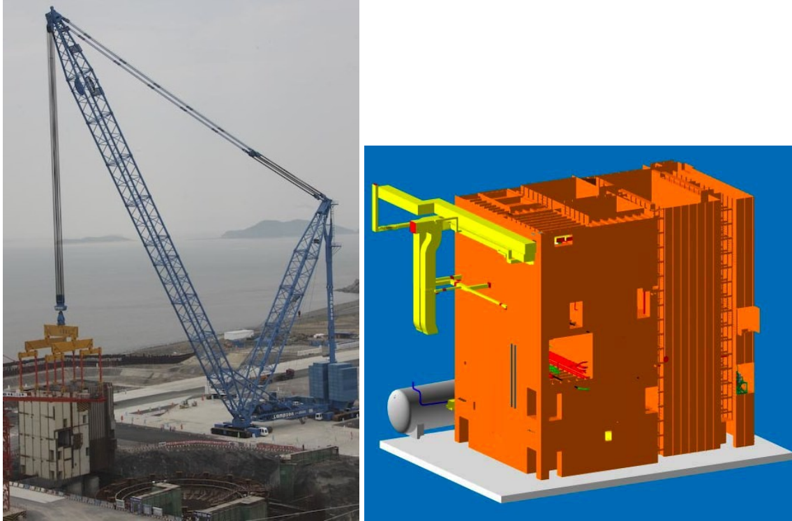
Fig. 11 An example of steel-plate concrete construction, a ~20-m high AP-1000 auxiliary building is assembled from factory-prefabricated modules and is set in place by a heavy lift crane in Sanmen, China (Credit Westinghouse).
