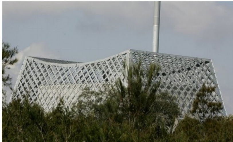
Fig. 1. External event shell steel grillage surrounds the Lucas Heights reactor in Australia.
