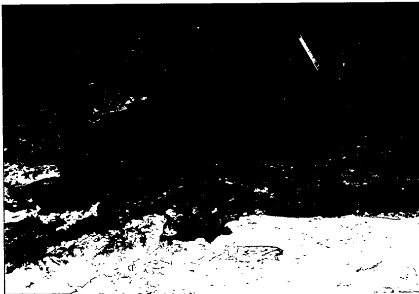
The appearance and chemical mixture in each tank depends on how the waste was generated and later waste management practices such as liquid evaporation, radionuclide removal, and waste mixing between tanks. This is a photograph of the surface of waste found in Hanford double-shell tank 241-101-SY. The steel pipe was bent during past waste movement during a gas release ("burp").
