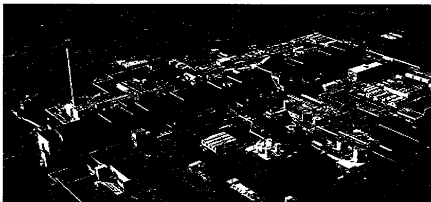
The PUREX Plant operated from more than 20 years, separating out plutonium and uranium from other materials using solvent extraction with the organic compound tributyl phosphate mixed in kerosene. The PUREX Plant is about 1000 feet long.
