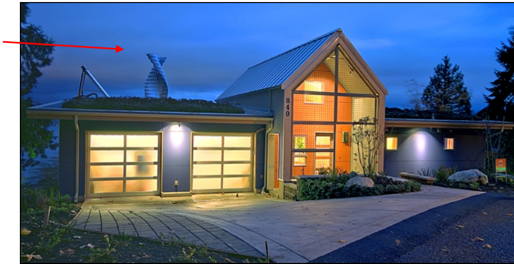
Figure 71: Shirey Zero Energy Idea House with evacuated tube panels on left
