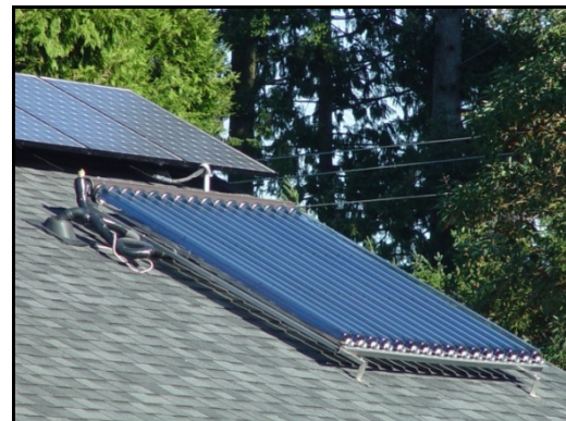
Figure 59. Martha Rose Construction SDHW systems
