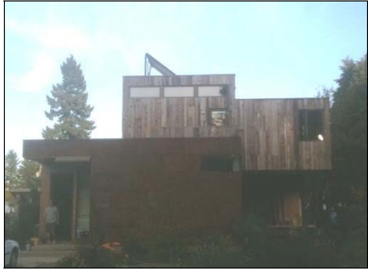
Figure 68. Solar panel tilted on flat roof
