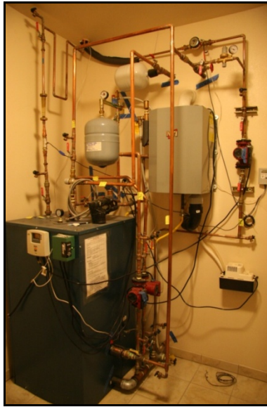
Figure 63. Solar thermal piping installation at Homestead
