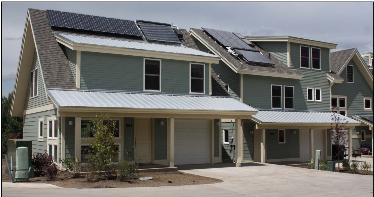
Figure 98. Snow Creek Cottages, Unit 10 (left) and 11 (right) with PV and Evacuated Tube Solar Hot Water
