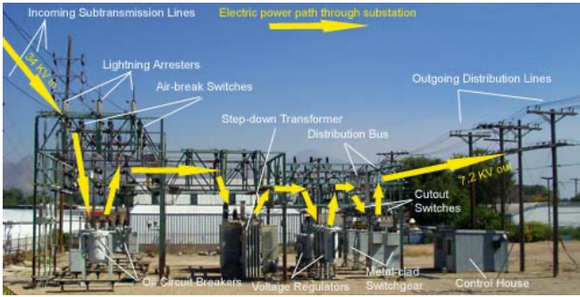
Fig. 5: Energy flow in a generic electrical substation.
