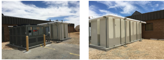
Figure 7. Latent heat storage system for heating/cooling peak load shifting [25].
