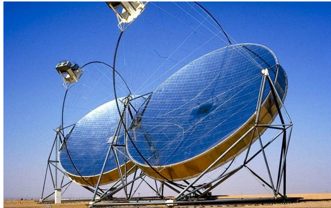
Figure 18. The SBP 17 m diameter stretched membrane dishes in Saudi Arabia [92].
