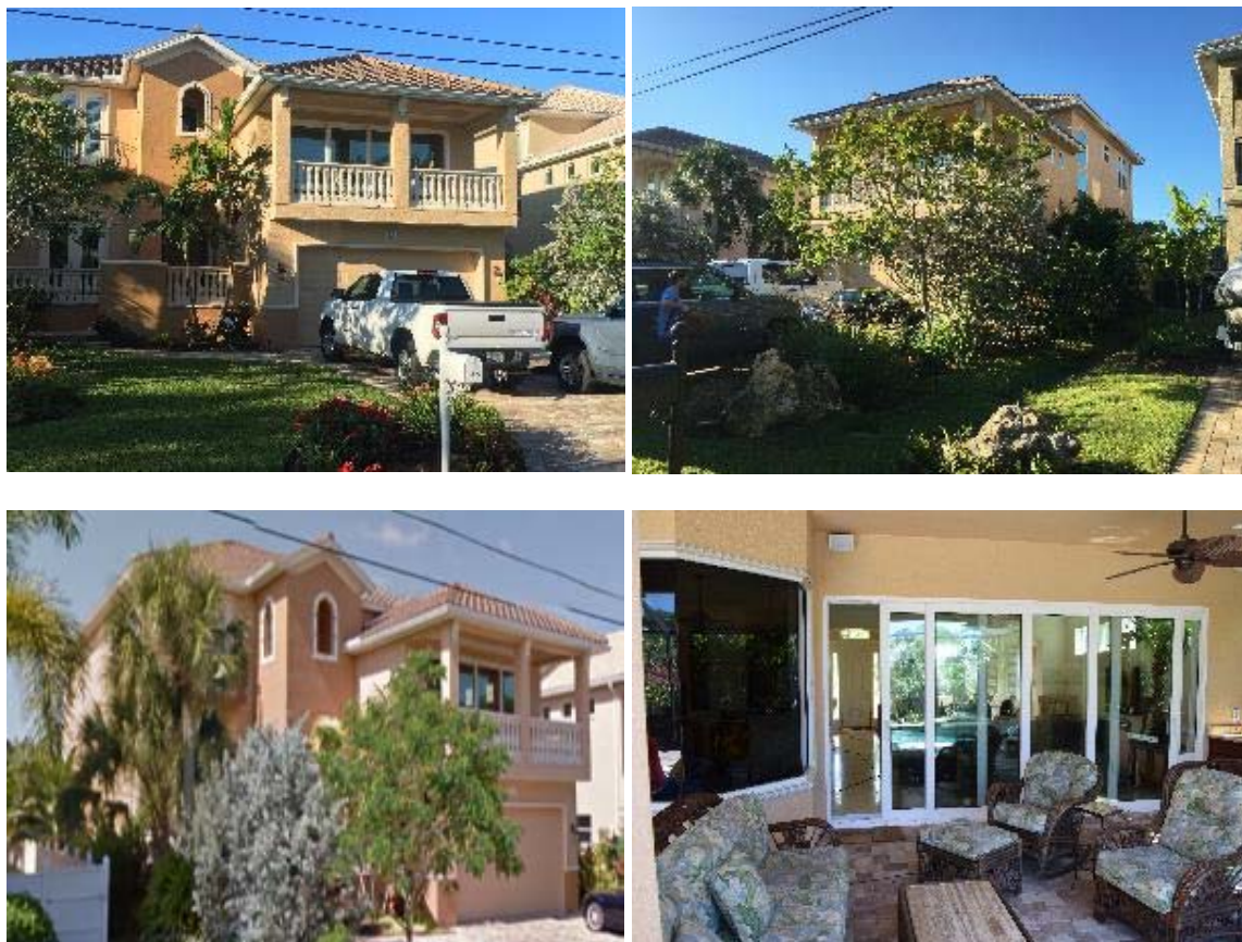
Figure 8: House 2 in Venice, FL
