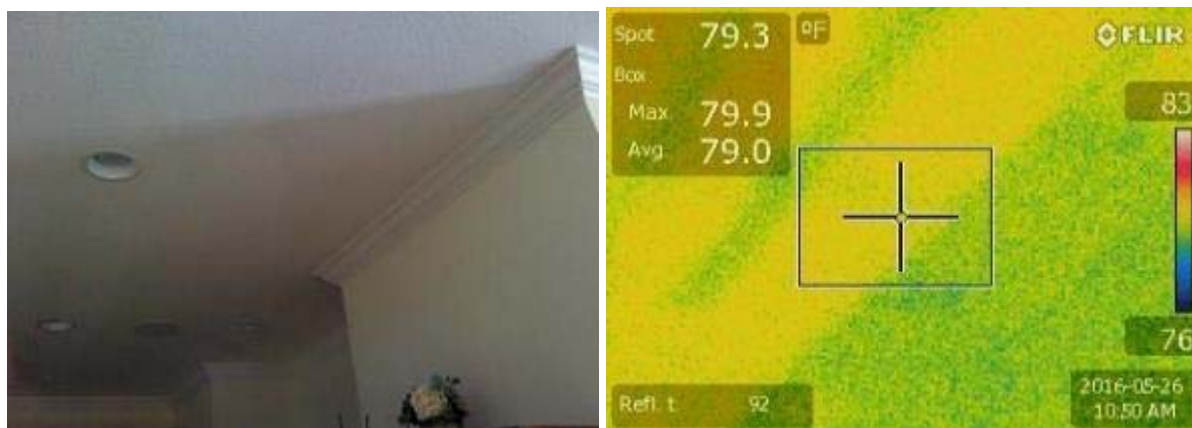
Figure 9: Digital and Infrared pictures of the attic under the South-facing roof
