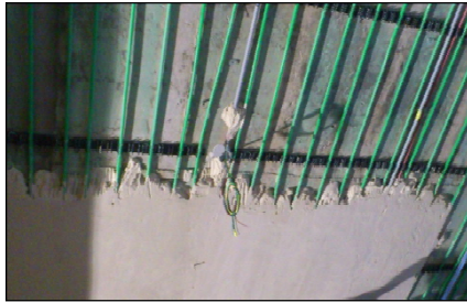
Figure 3: Radiant ceiling cooling system
