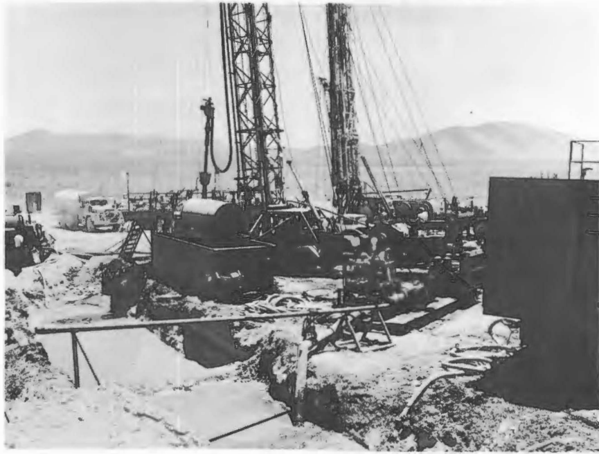
Figure 5 - PUTTING RADIOACTIVE SAMPLES DOWN HOLE
