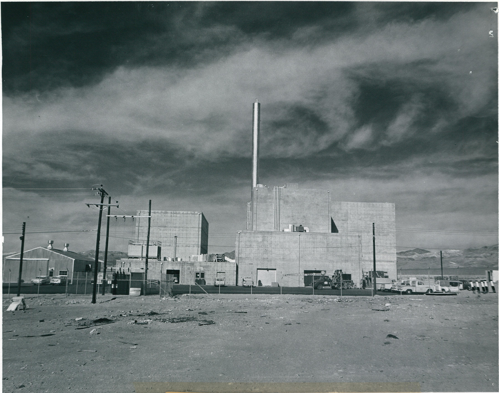
ALO-LVB - MAD Building, Looking North Sierra Construction Corporation Contract AT (29-2)-628 25 January 1959
